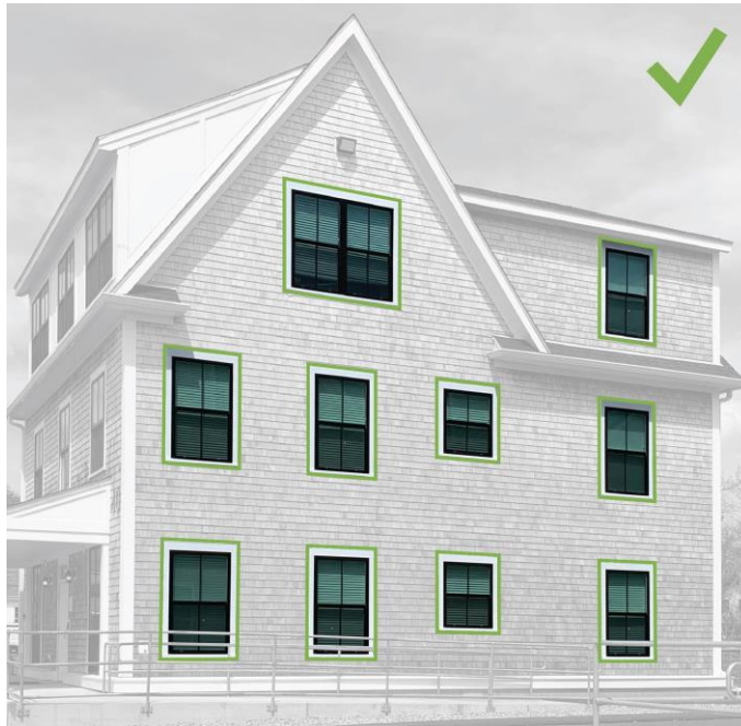
Figure 10: Example of two-over-two sash windows with an exterior muntin
