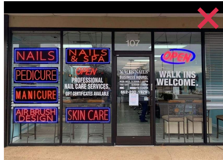
Figure 38: Example of signage that obscures windows and architectural features
