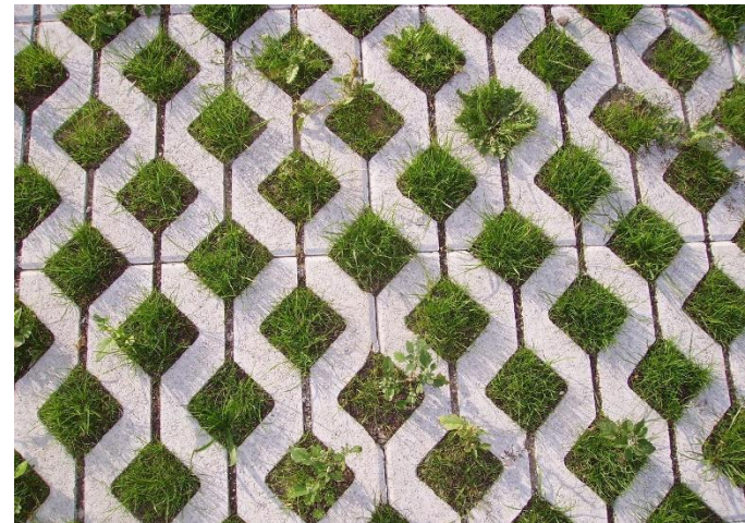
Figure 17: Example of pervious materials for parking lots
