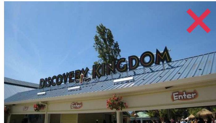
Figure 42: Example of wall sign that is inappropriately mounted on a track and not recommended.
